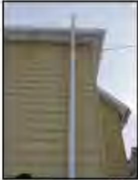
The vent pipe is routed **up** the side of the structure to a location above the roof line.
