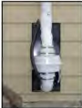
A fan is used to draw soil vapor from beneath the slab.
