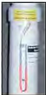
A liquid gauge, or manometer is used to verify that the system is operating properly
